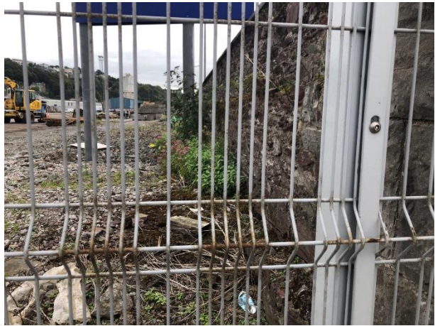
Photo 4. Works yard located next to Horgan's Quay
