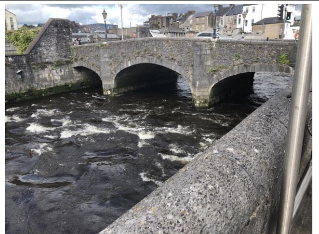
Photo 12. South Gate Bridge from French's Quay STC G Togher to City
