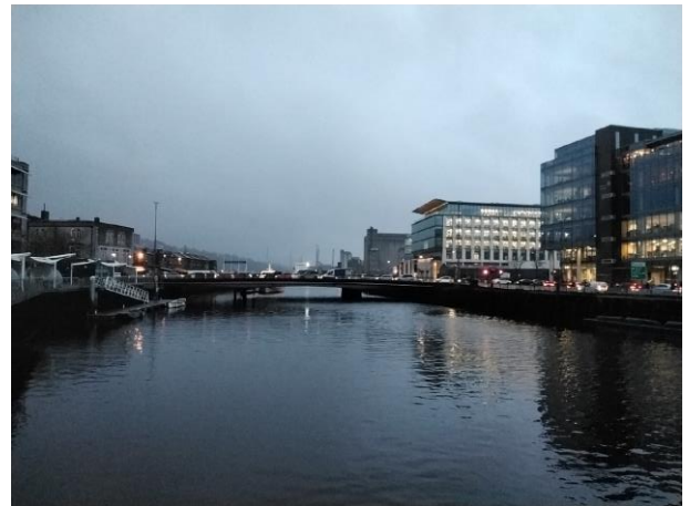
Photo 20. River Lee looking east from Clontarf Bridge
